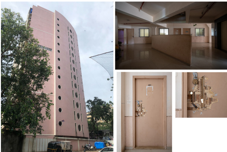
Figure 2. Diamond Apartments, the Slum Rehabilitation building in Mumbai and its alienating environment, where one of the walls on the building facing a so-called "sale building" is kept blank so as to conceal their presence. Photo by Rupali Gupte.
